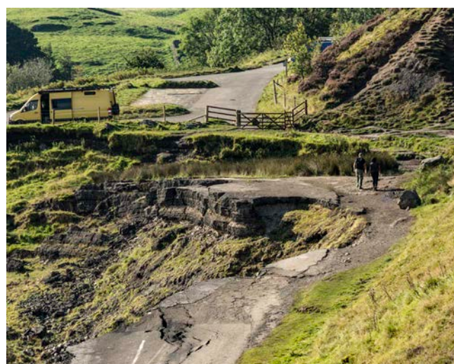
Figure 8. The abandoned road across the Mam Tor landslide, as it appeared during 2020, with slices continuing to fall away where it is underlain by the complex slide structure.
