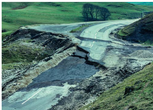
Figure 7. The upper road onto the Mam Tor landslide, the day after it was broken in 1977 by movement of the small rotational slide within the main slide mass.
