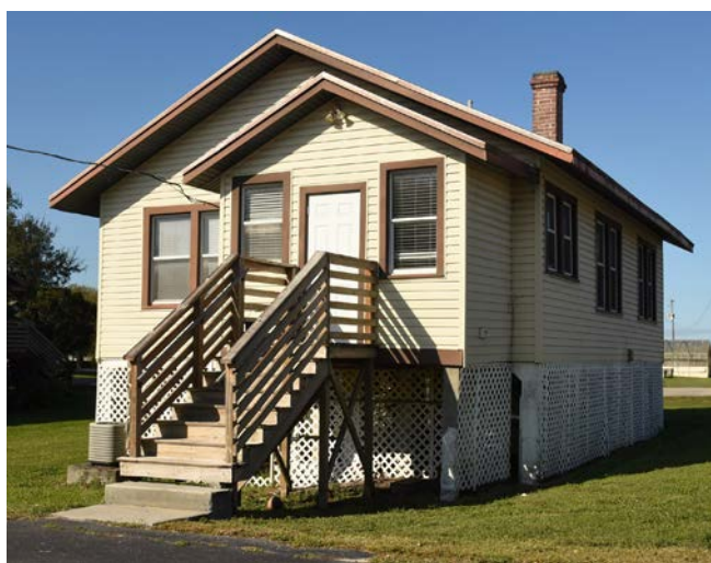
Figure 4. A house at Belle Glade university site, which was close to ground level when built in the early 1950s.
